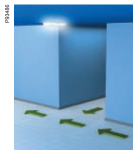
At every corridor intersection.
